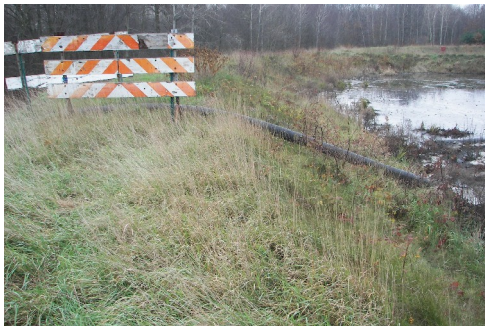
Pipe carrying dredgings going to the containment pond
